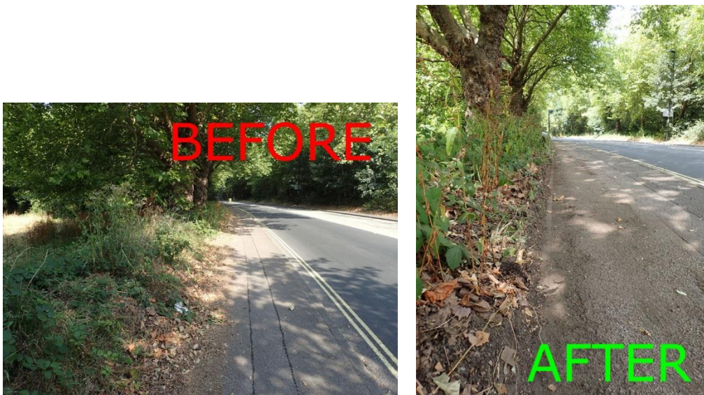
Highfield Avenue, lost pavement – Photos July 2018
